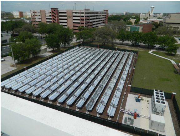
CERC's concentrating solar thermal pilot power plant as R+D tool and teaching vehicle.
