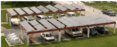
CERC's 20,000 watt solar / electric charging station at the USF in Tampa.
