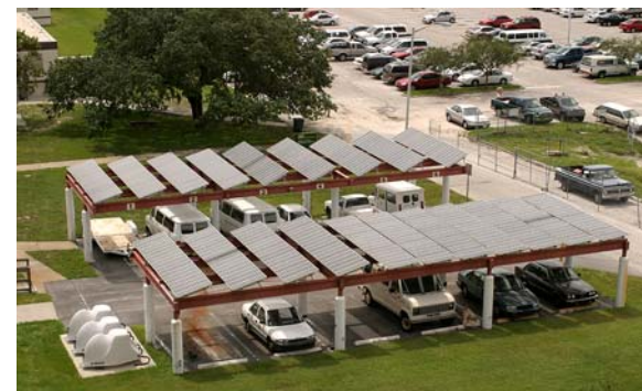
The solar energy charging station, designed, developed and built by CERC consists of a parking/charging facility for 12 electric vehicles providing up to 20 kilowatts of peak power.
