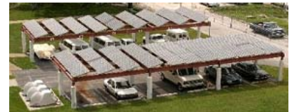
20,000 watt solar/electric charging station
