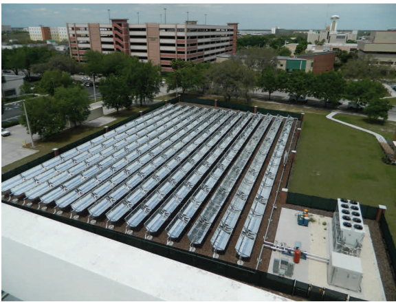
CERC's concentrating solar thermal pilot power plant as R+D tool and teaching vehicle.
