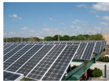
The original CERC PV array generated 20 kW of electricity. Presently, half of the system is being renovated with new PV modules to provide 10kW of electricity to be tied to the utility grid.
