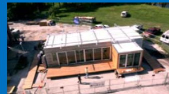
USF's Flex House during construction.
