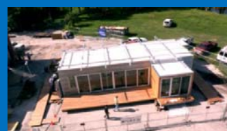
USF's Flex House during construction.
