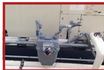
Refrigerant flow meters wired and connected to data logger system.
